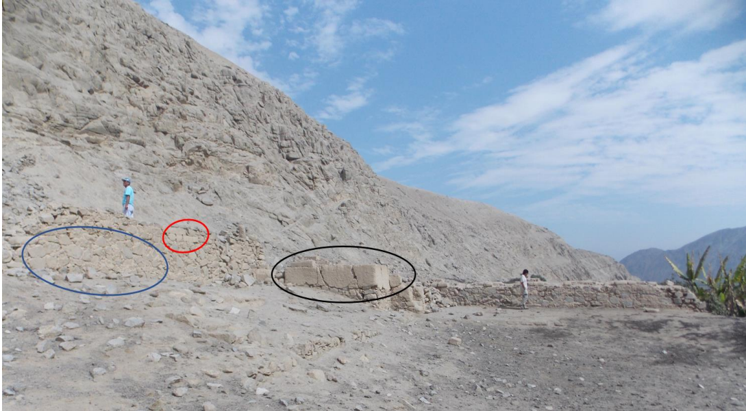
Figure 5-8 Ruined structures at the site of Escalón in Lunahuaná. Note the presence of three construction techniques: (a) field stone and mud mortar (b) adobe (c) tapia.
