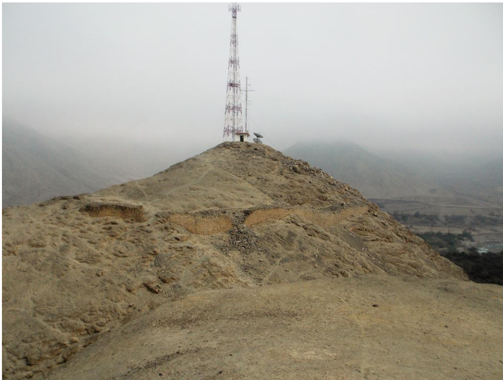
Figure 4-4 Massive curtain wall surrounding the peak of Cerro Pascua. A modern cellular tower corroborates the favorable vantage.
