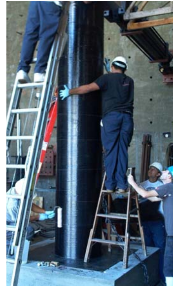
Figure 2-23: Shell Construction
