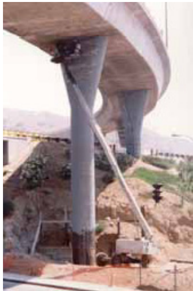
Figure 1-9: Welding of Steel Jacket for a Caltrans Strengthening Project [26]
