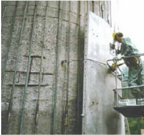
Figure 1-11: Installation of a Pre-Cast Concrete Shell Jacket [26]
