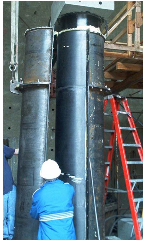
Figure 2-29: Removal of Steel Mold
