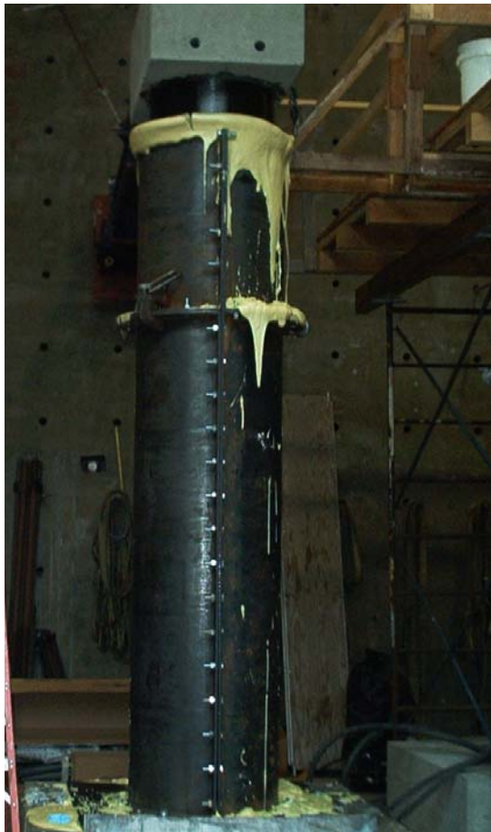
Figure 2-28: Curing of Jacket
