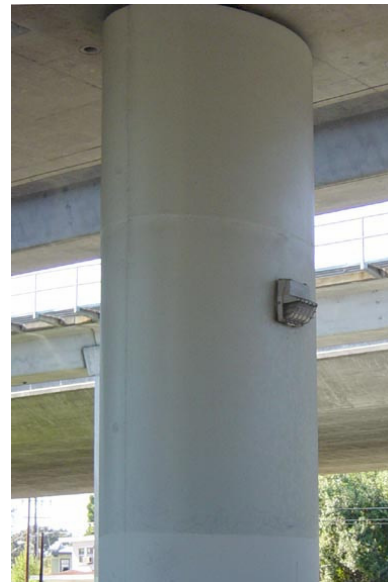
Figure 1-10: Completed Steel Jacket Column Retrofit [27]
