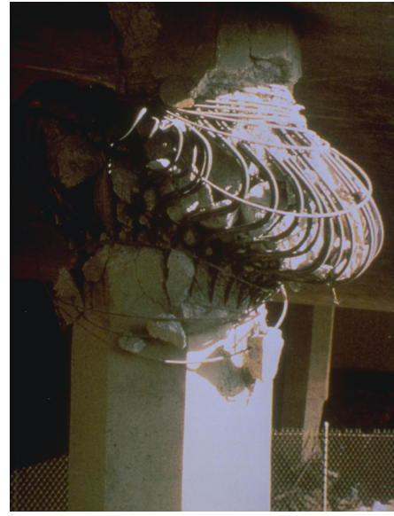
Figure 1-16: Lack of Confinement Failure [37] Figure 1-17: Lack of Confinement Failure [37]
