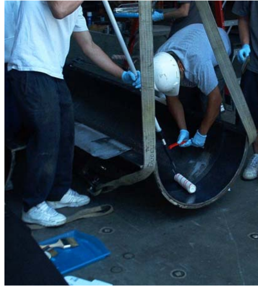
Figure 2-20: Placement of Carbon Fabric
