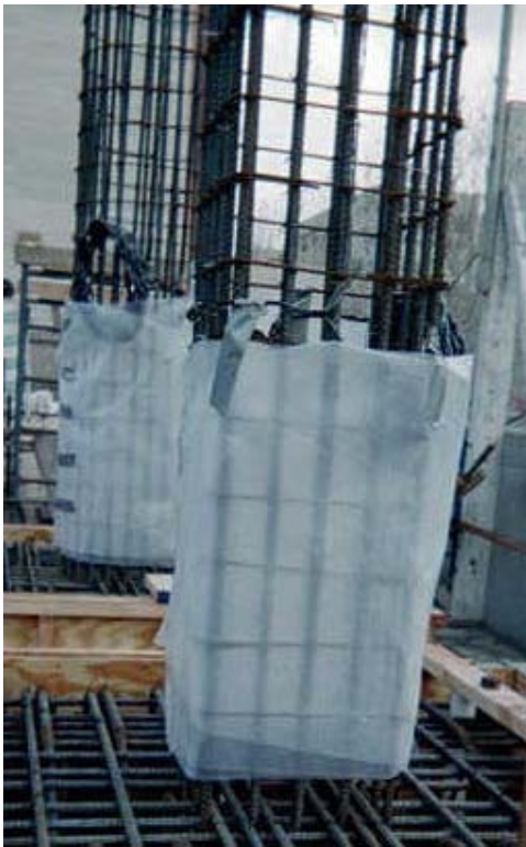
Figure 3-3: Shear Column Cages
