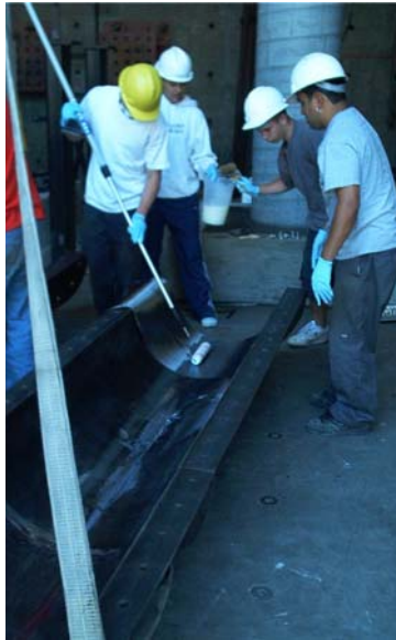
Figure 2-21: Jacket Construction
