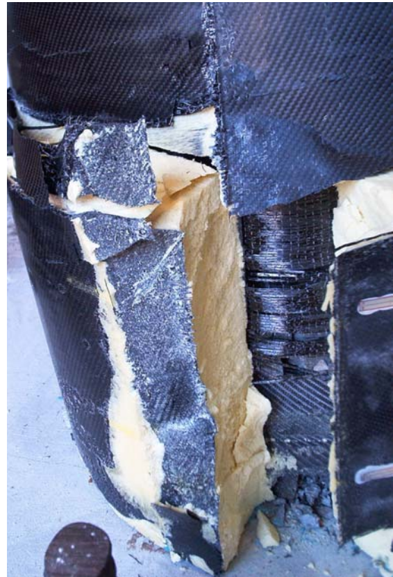
Figure 4-52: Close up of Jacket Failure
