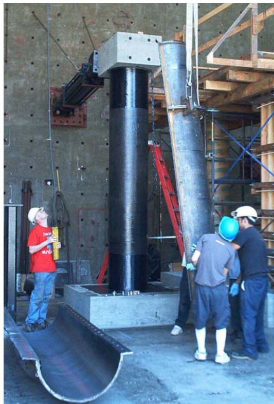
Figure 2-24: Placement of Steel Mold
