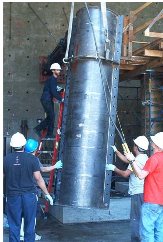
Figure 2-25: Placement of Steel Mold
