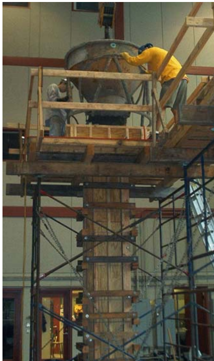
Figure 3-7: Shear Column Concrete Placement
