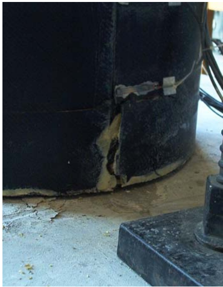
Figure 5-45: Jacket Splitting at Seam
