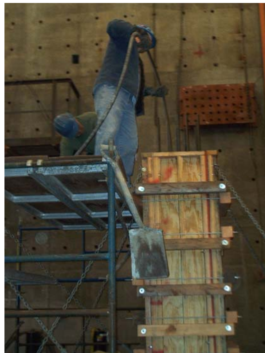
Figure 3-8: Vibrating Shear Column Concrete for proper consolidation
