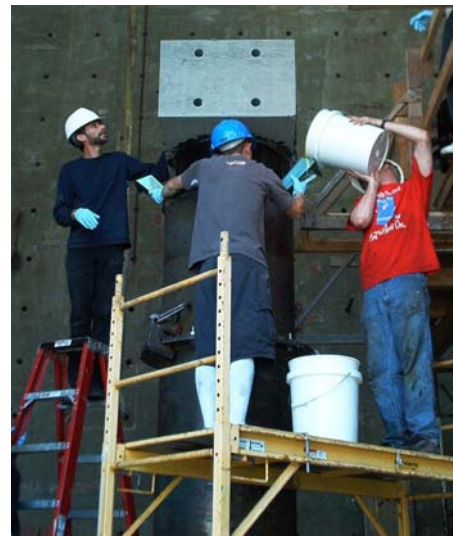
Figure 2-26: Lapping of the Jacket Seams Figure 2-27: Pouring of Expandable Foam Core
