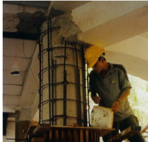
Figure 1-12: Installation of Poured- in-Place Concrete Retrofit Jacket [29]
