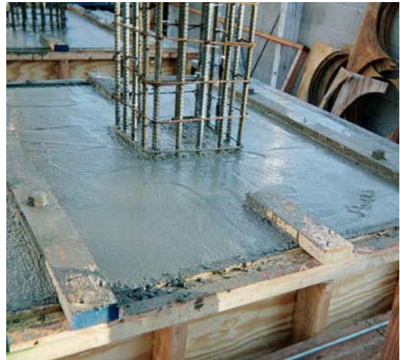
Figure 3-6: Finished Column Base Concrete
