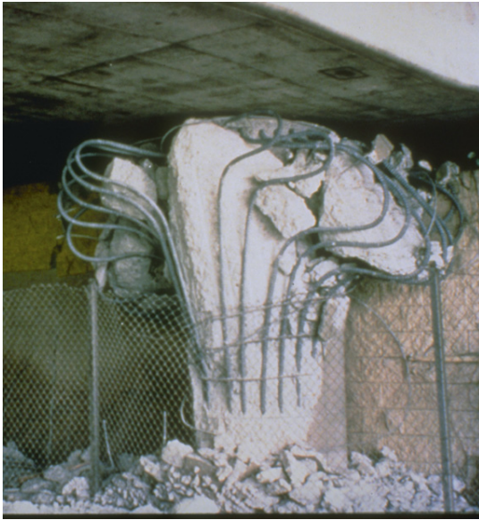
Figure 1-16: Lack of Confinement Failure [37] Figure 1-17: Lack of Confinement Failure [37]
