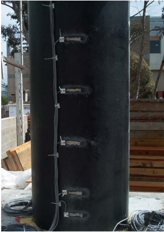
Figure 3-11: Jacket Gages at Located at North Load Face of Shear Column
