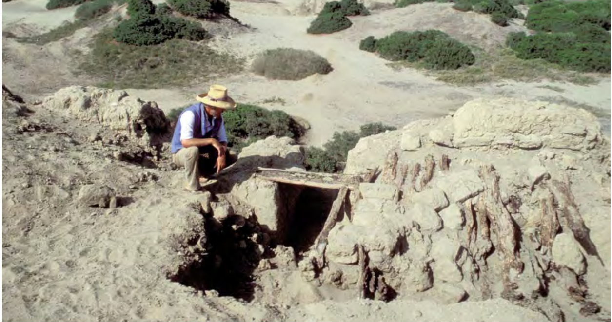
Figure 15 The subterranean corridors being exposed. Note the lintel in place above one of the windows, and the beams spanning the top of the corridor.
