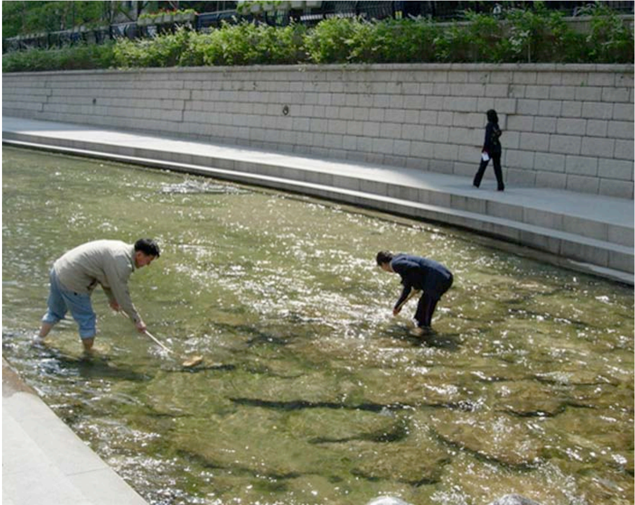
Figure 27. Workers scrub the algae off the rocks and bottom of the Cheonggyecheon (François Rejeté).
