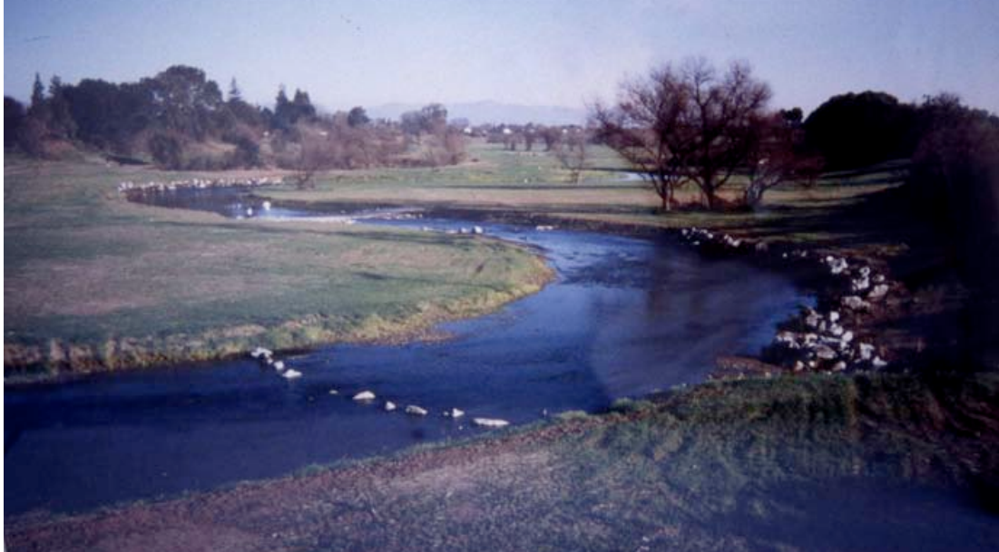
Figure 13. Uvas Creek restoration with armoring on the outside of the bends and rock weirs spanning the channel in January 1996, two months after construction (City of Gilroy, from Kondolf 2006).
