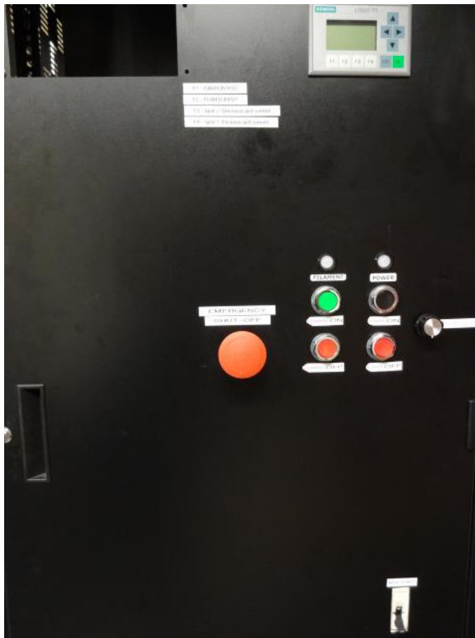
Fig. 12 – Front panel of power supply. All screens, buttons, knobs, and switches are labeled.
