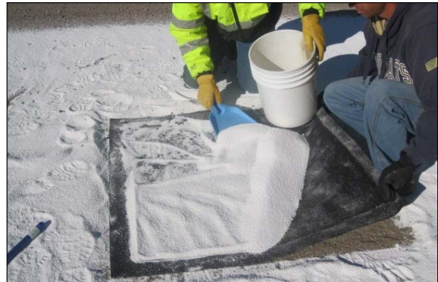
Figure 5.15: Checking application rate of calcium chloride flakes.
