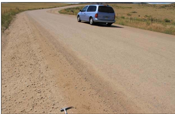
Figure 3.1: Good gravel road.
