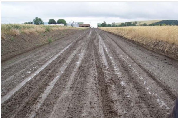
Figure 1.3: Impassability in wet weather.
