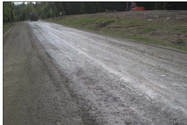
Figure 5.12: Good penetration with pre-wetting.
