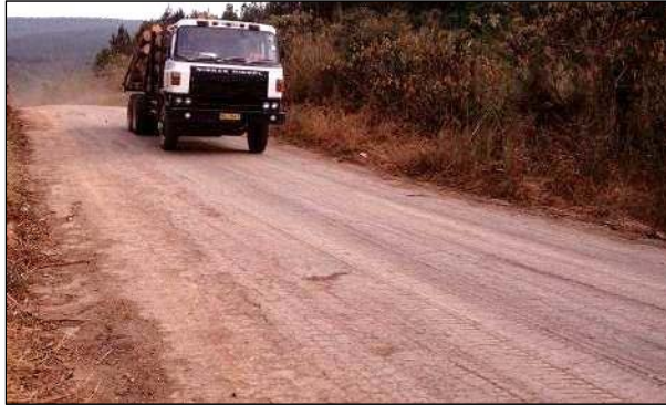
Figure 2.11: Road treated with concentrated liquid stabilizer.
