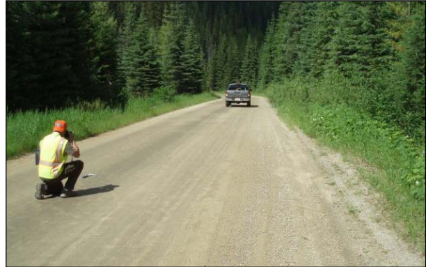
Figure 2.4: Road treated with magnesium chloride.
