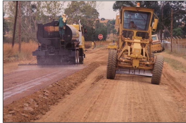
Figure 5.25: Blade mixing application.
