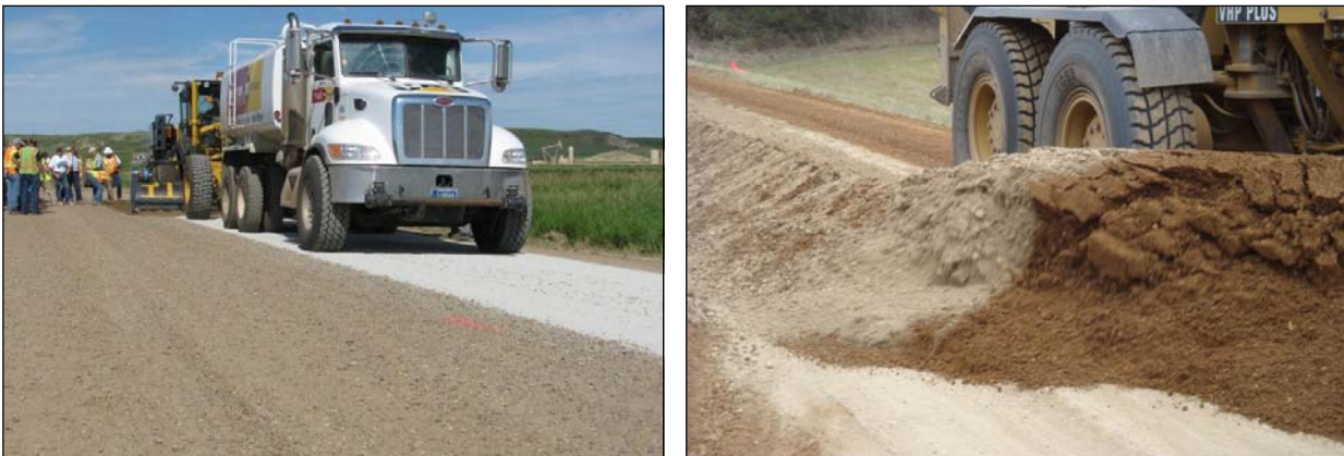
Figure 2.12: Mechanical stabilization with bentonite.
