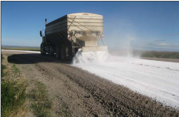
Figure 5.14: Flake application of calcium chloride.
