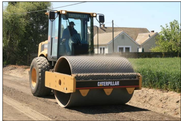
Figure 5.21: Compaction with a smooth-drum roller.
