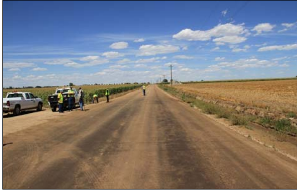
Figure 2.6: Road treated with lignosulfonate.
