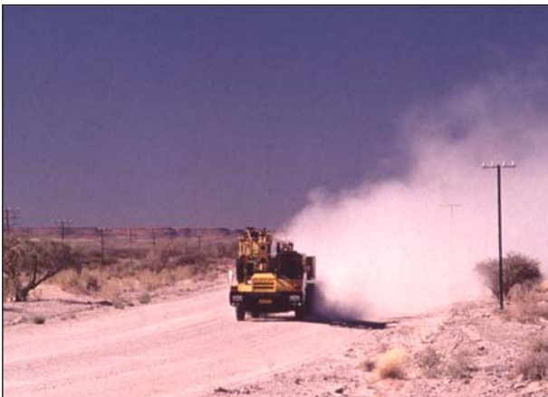
Figure 1.1: Unacceptable levels of dust.
