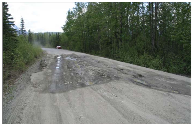
Figure 1.3: Impassability in wet weather.
