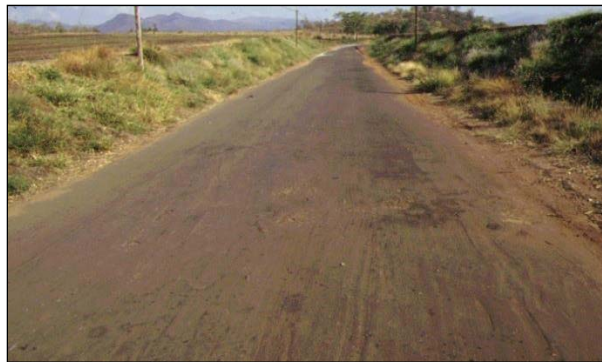
Figure 2.7: Road treated with asphalt emulsion.
