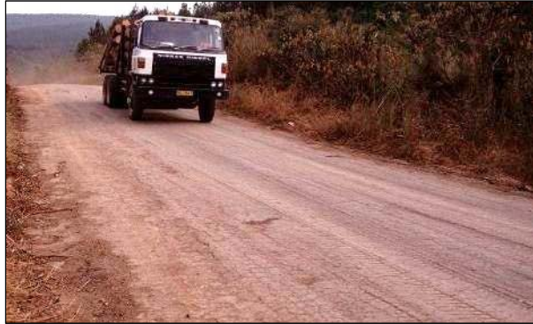
Figure 2.11: Road treated with concentrated liquid stabilizer.
