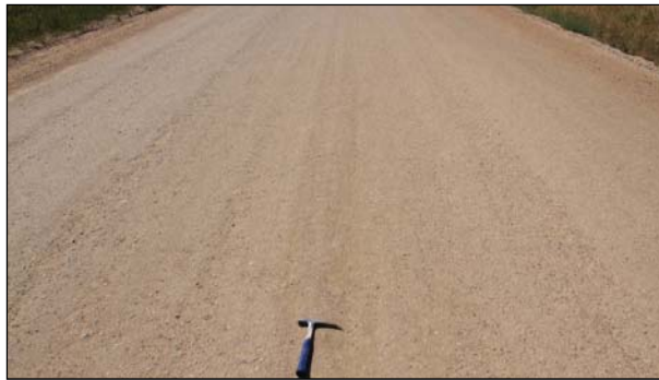
Figure 2.10: Road treated with synthetic polymer emulsion.
