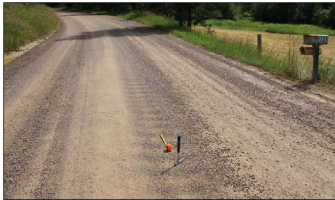
Figure 5.3: Poor performance after treatment application to a poorly prepared road (loose gravel).
