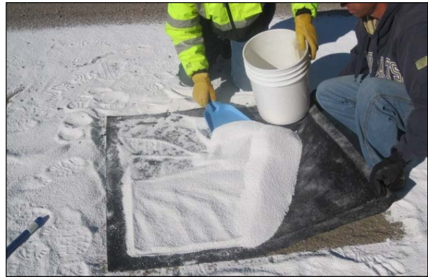
Figure 5.15: Checking application rate of calcium chloride flakes.
