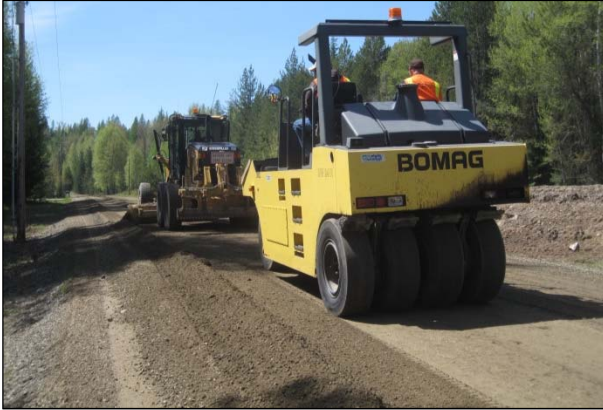
Figure 5.22: Compaction with a rubber-tired roller.
