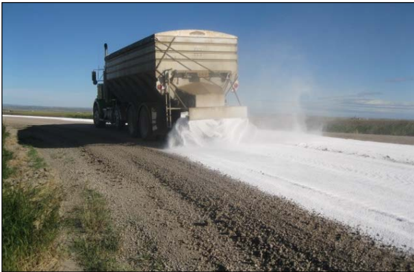
Figure 5.14: Flake application of calcium chloride.
