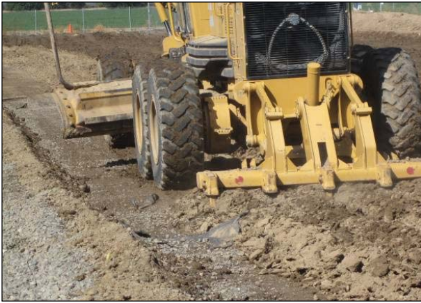
Figure 5.18: Ripping with a grader.
