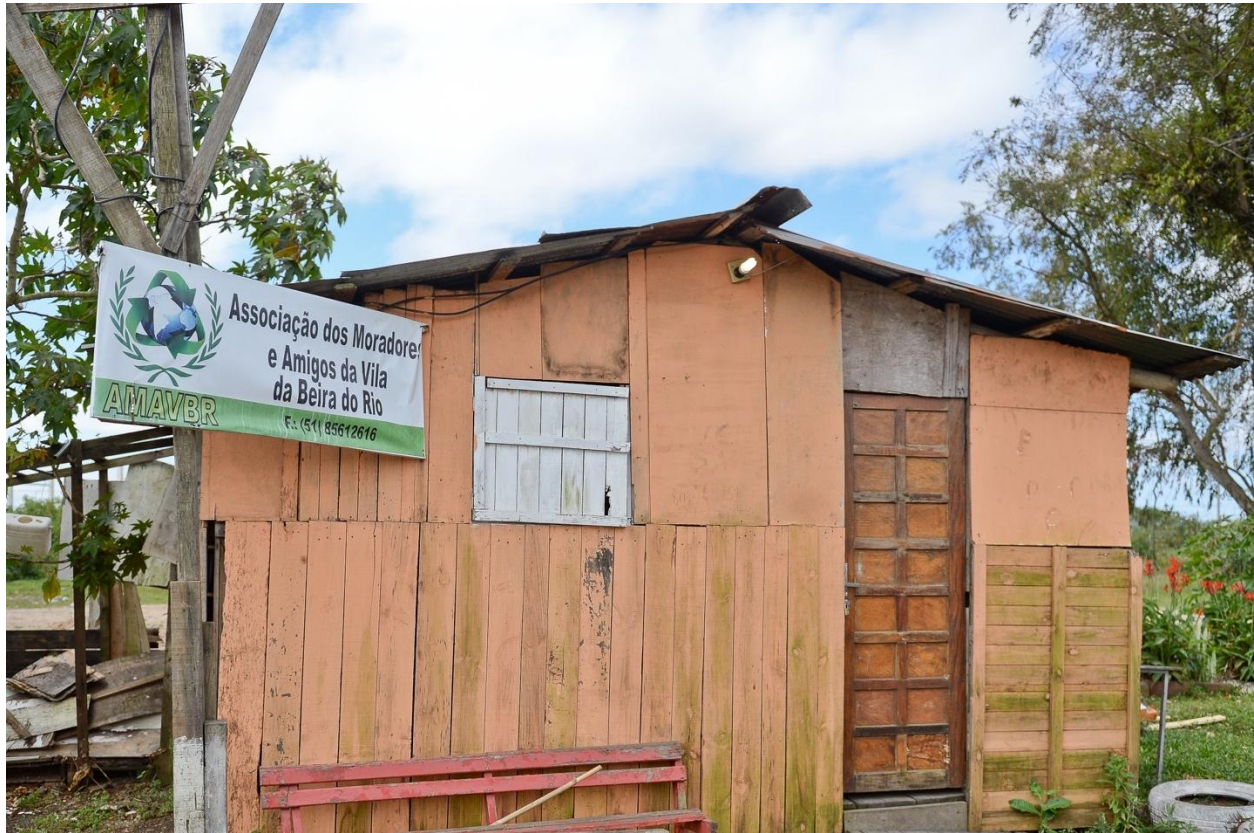
Figure 37: Shed at Vila da Beira do Rio’s Friends and Residents Association in Porto Alegre Source: Josieli Silva/CMPA
