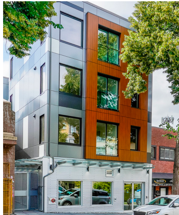
Figure 8. 10-Unit Building on 3,400 Sq. Ft. Lot in Vancouver, British Columbia
