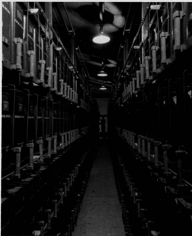
FIG. 9 ONE SECTION OF CAPACITOR BANK
