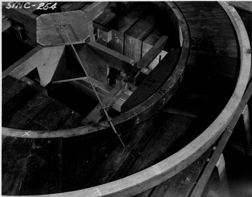
POLE BASE WEDGE CIRCLE NEARLY COMPLETE
