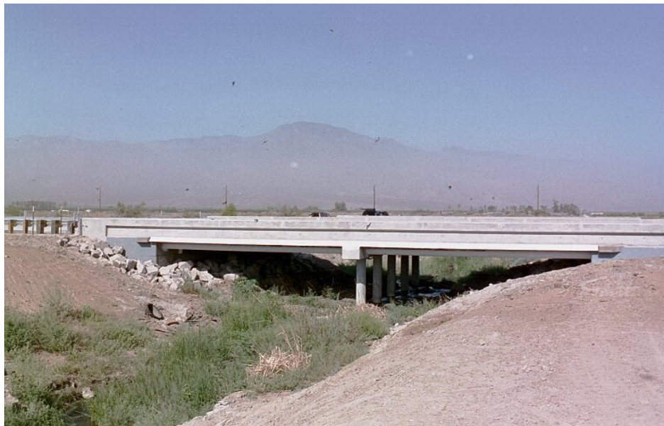
Figure 6-1 Kings Stormwater Channel Composite Bridge
