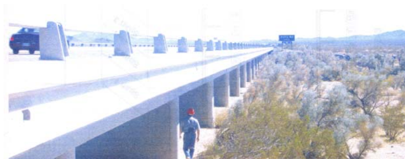
Figure 3-8 Aerial Photo of the Watson Wash Bridge
