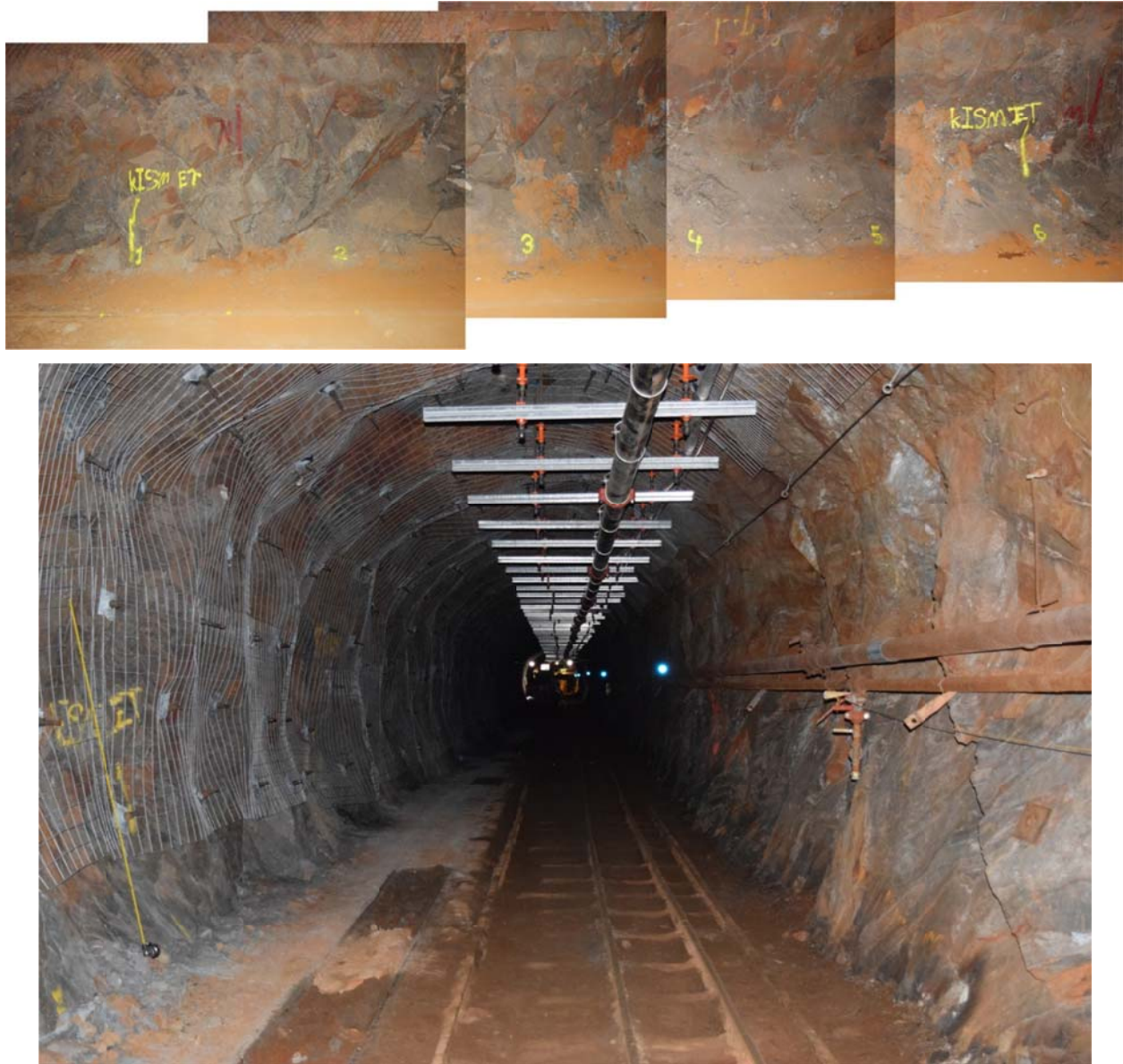
Figure 2.10. Upper image: Composite photo of site taken on May 21, 2015 spanning approximately 60 ft (18.3 m) along the east rib of the West Access Drift. Lower image: Photo taken in February 2016 showing new ground support consisting of rock bolts and wire mesh. (For reference, the yellow kISMET spray paint on right-hand side of upper image is the same as that in left-hand side of lower image.).
