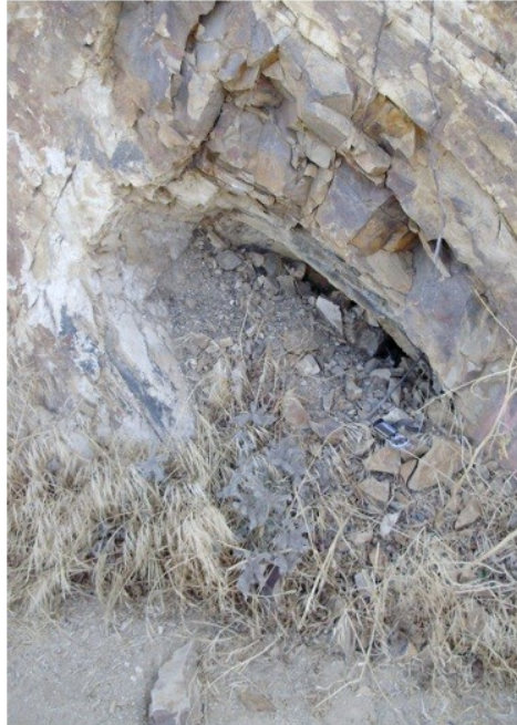
Figure 16. View of the small cave along the Lower Beacon Trail of Griffith Park, where three faults converge. The camera is facing SW, and a Silva Ranger transit is open in front of the cave, on the right, for scale (Helman, 2009c).
