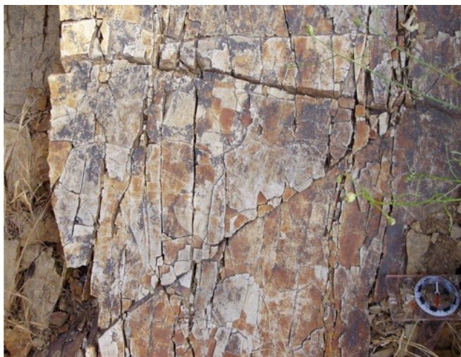
Figure 8. Jointing along the Lower Beacon Trail in Griffith Park. The two prominent joints form a 60° angle. The Silva Ranger Transit in the corner is here for scale (Helman, 2009b).
