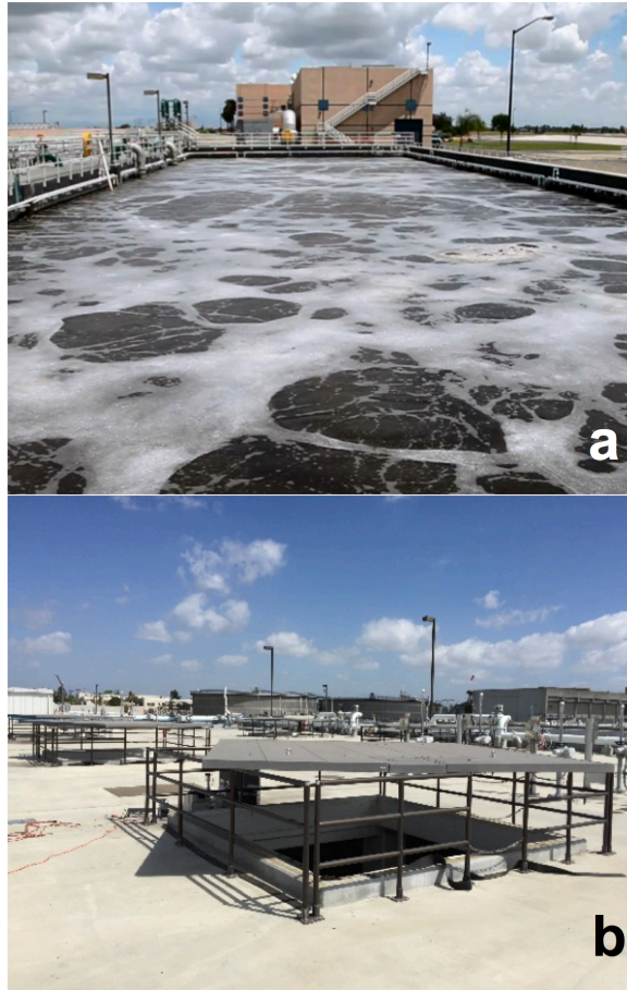
Figure 3-1: Pictures of a) an open aerated basin and b) a semi-covered aerated basin at Orange County Sanitation District (OCSD). The open basin allows all particulates to escape into the atmosphere while the semi-covered basin may reduce a small portion of particulate emissions due to particle impaction on the basin ceiling. Figure 3-1a source: Marnette Federis (Public Radio International).
