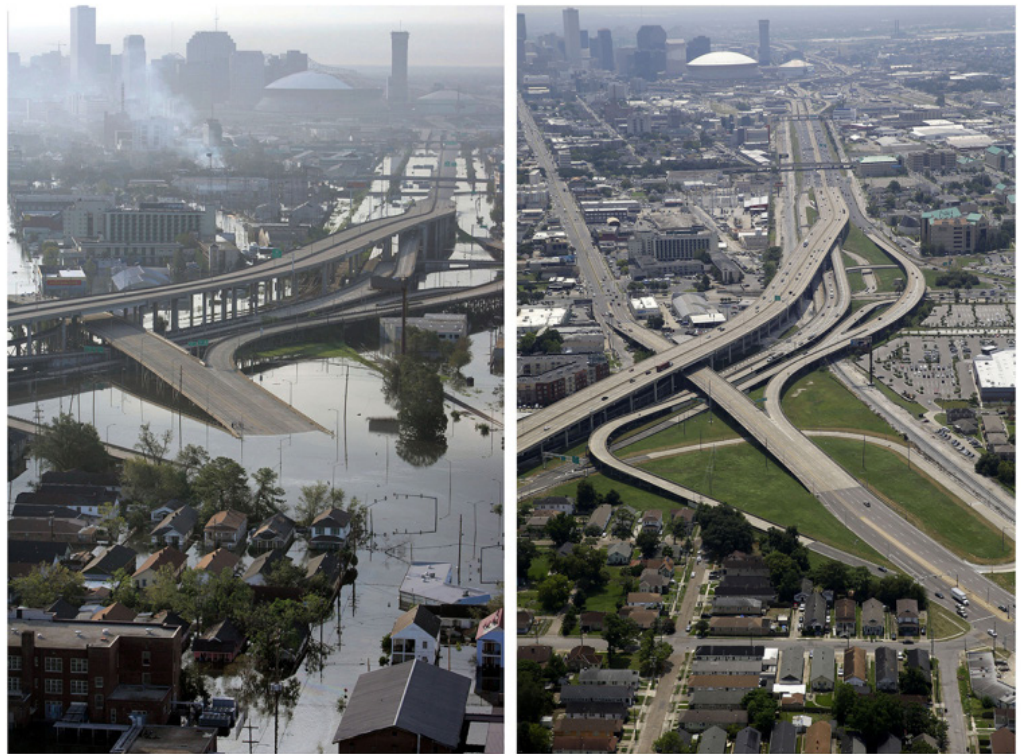
I-10 HIGHWAY DURING AND AFTER HURRICANE KATRINA.
