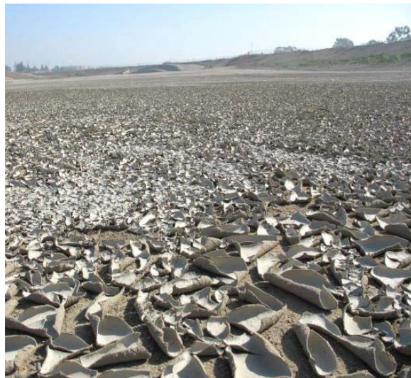
Figure 20: Accumulated clogging layer from a recharge basin operated by OCWD (from Figure 5-12 [26]).
