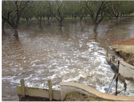
Figure 7: Application of storm water on an almond orchard for groundwater recharge.
