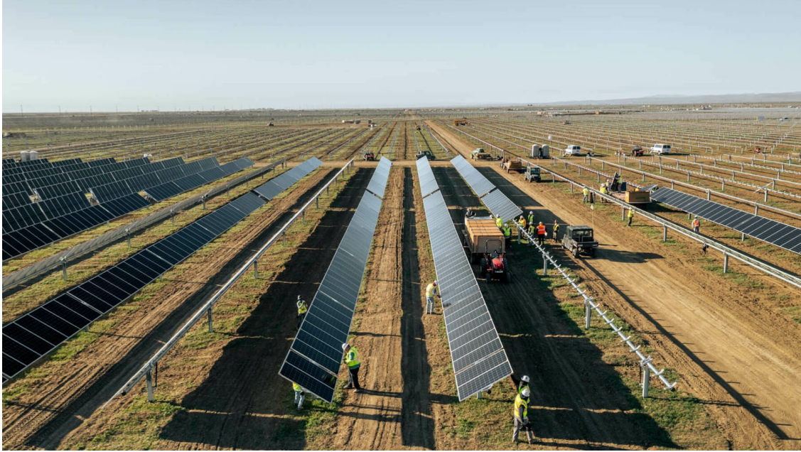
Figure 5: Lifting glass at Westlands Solar Park, Aquamarine branch. (SOLV Energy, 2021)
