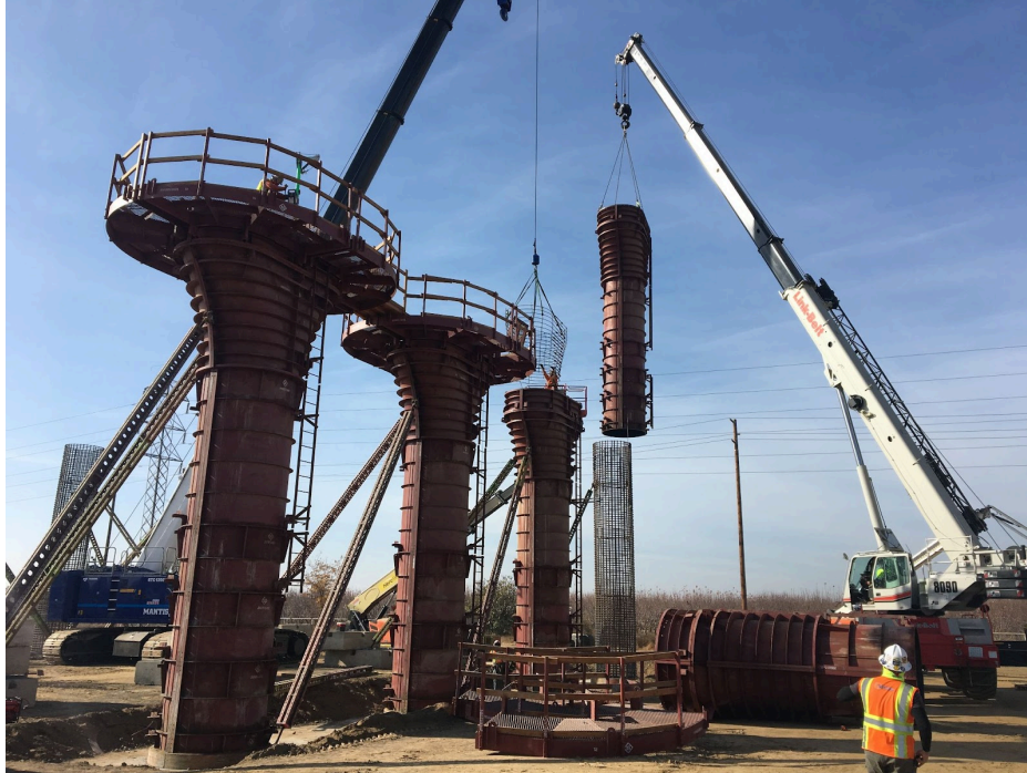
Figure 6: Raising high speed rail platform towers, near Hanford, CA. (Author, 2020)
