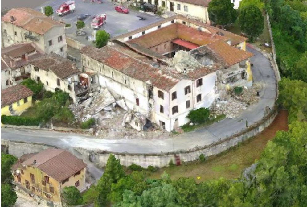
Figure 5.3. Excerpt of the 3D model with the most damaged portion of Accumoli (easternmost part of the village).
