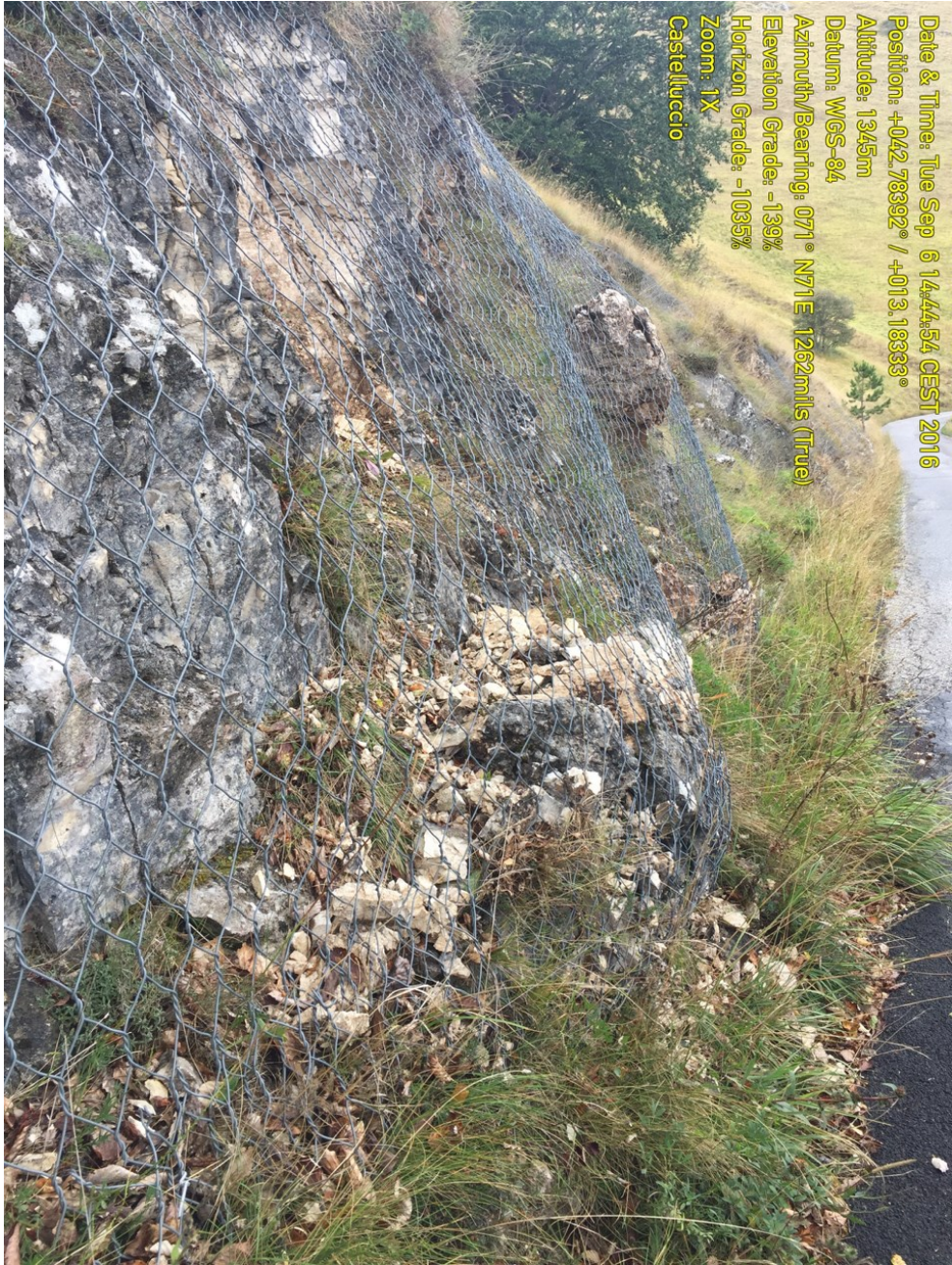
Figure 4.20. Rock-net protection with captured debris from the earthquake, including minor small debris in the foreground and a large ~0.5-m block in the background (42.78392 N 13.18333 E).
