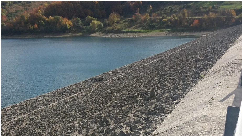
Figure 7.15. Poggio Cancelli embankment dam on the Campotosto reservoir (L'Aquila): photo of the upstream face taken on October 19, 2016 (42.557106°N, 13.338342°E).
