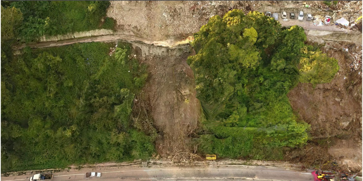
Figure 4.29. 3D model of smaller landslide adjacent to Highway SS4 (42.7501 N 13.2719 E).
