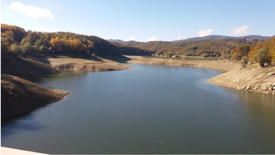
Figure 7.14. View of the reservoir from Scandarello dam viewpoint (October 19, 2016): no phenomena of bank instability were observed after the earthquake.
