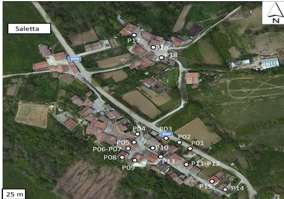
Figure 5.66. Locations of representative structures inspected in Saletta (see Table 5.17 for details).
