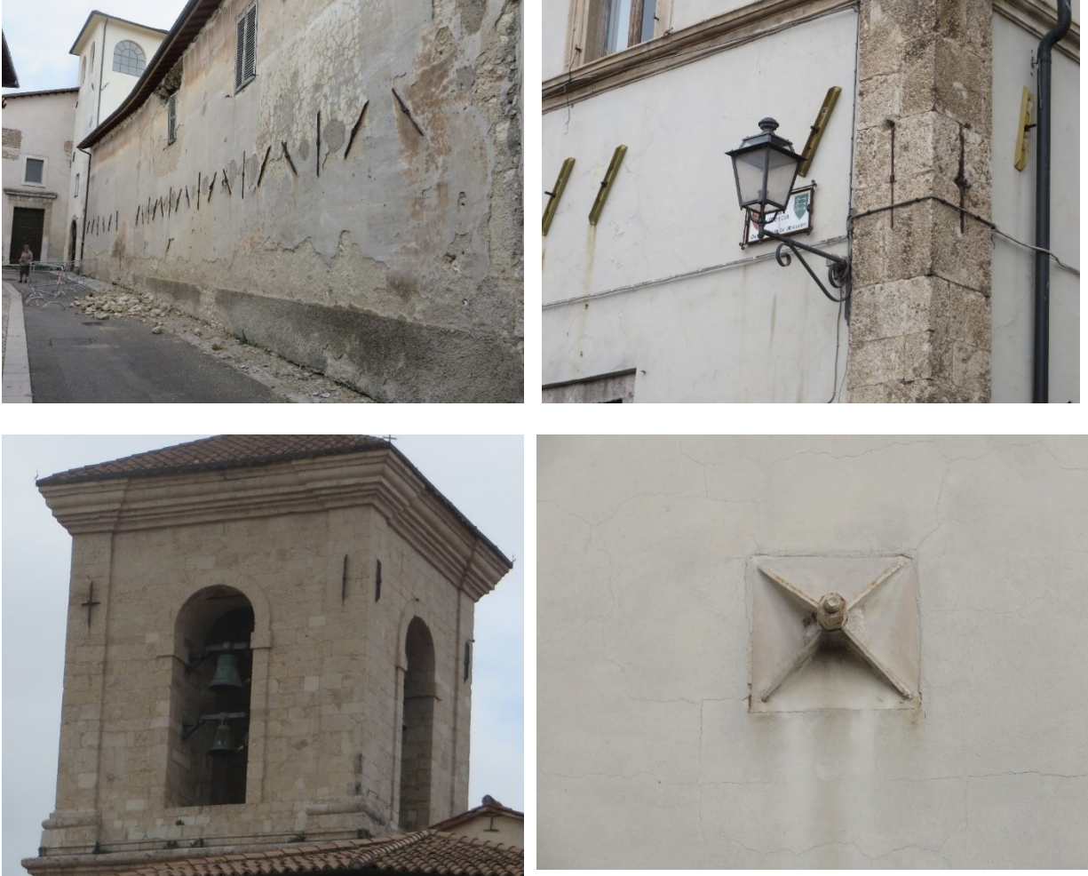
Figure 5.35. Buildings and towers retrofitted with cross-ties in Norcia.
