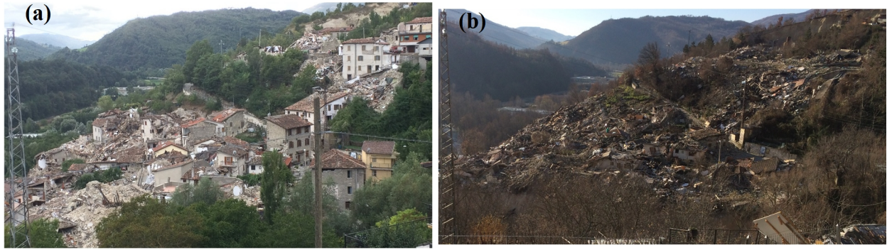
Figure 12. Incremental damage in Pescara del Tronto after the October earthquake events. (a) Overview of Pescara del Tronto on 9 September 2016, (b) Overview of Pescara del Tronto on 12 December 2016.
