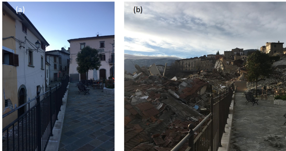
Figure 14. Incremental damage in Accumoli after the October earthquake events. (a) Overview of Accumoli, September 2016, (b) Overview of Accumoli December 2016.
