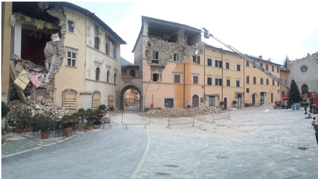
Figure 15. Damages observed in Piazza Martiri Vissani (Visso).
