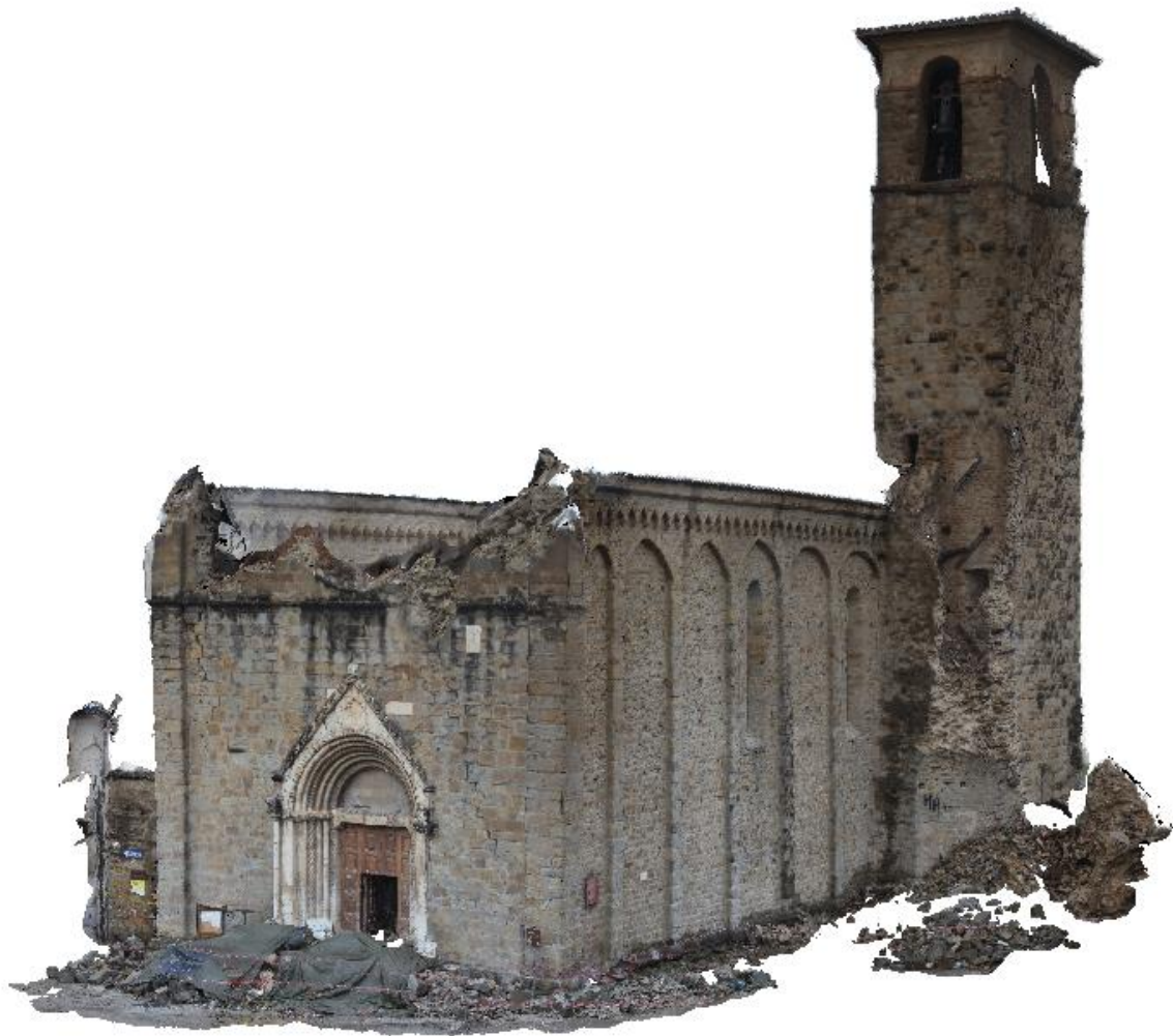
Figure 9. 3D textured model of the Sant'Agostino church and its bell tower in Amatrice. (N42.628, E13.2914, September 7 2016, Figure prepared by: F Chiabrando, V Di Pietra, and N Grasso).
